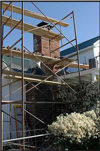
Putting in the flashing.
