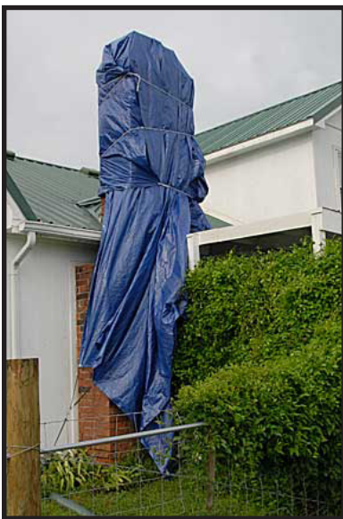
Tarped to minimize water seepage to basement.
