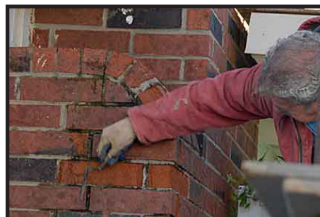
Removing the bad brick.
